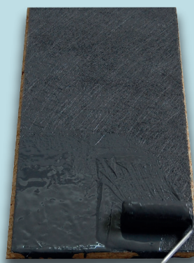
3. Apply second coat of Pro-Roof, ("wet on wet")
