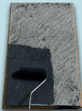
2. Apply Promesh 225 & Dry roll to embed.
